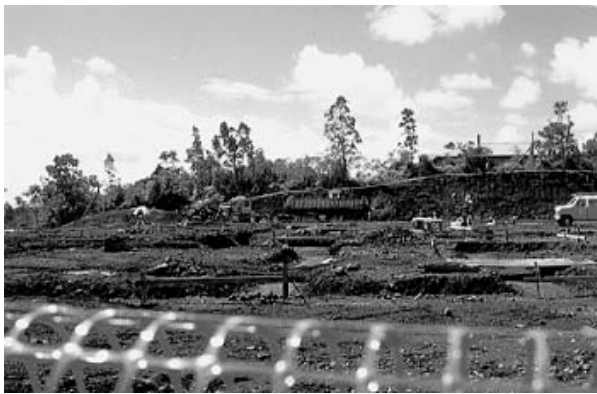
Figure 2. Hilo Base Facility construction, September 1997.
