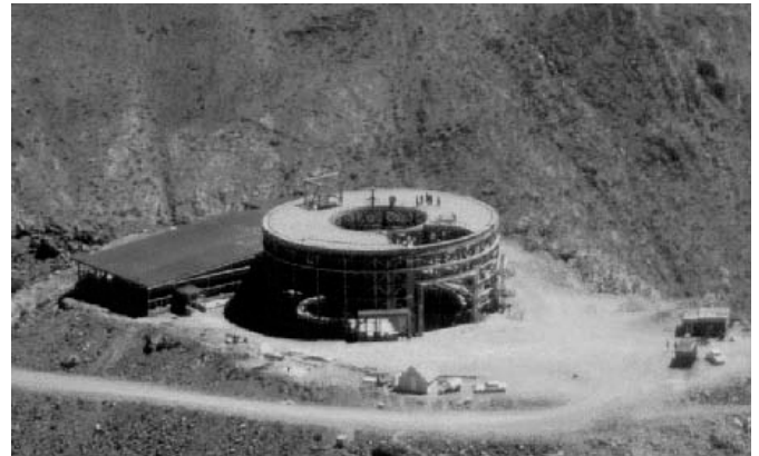
Cerro Pachon site construction in January 1997.
